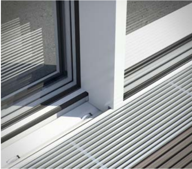
Detailansicht von außen Detailed view from outside
